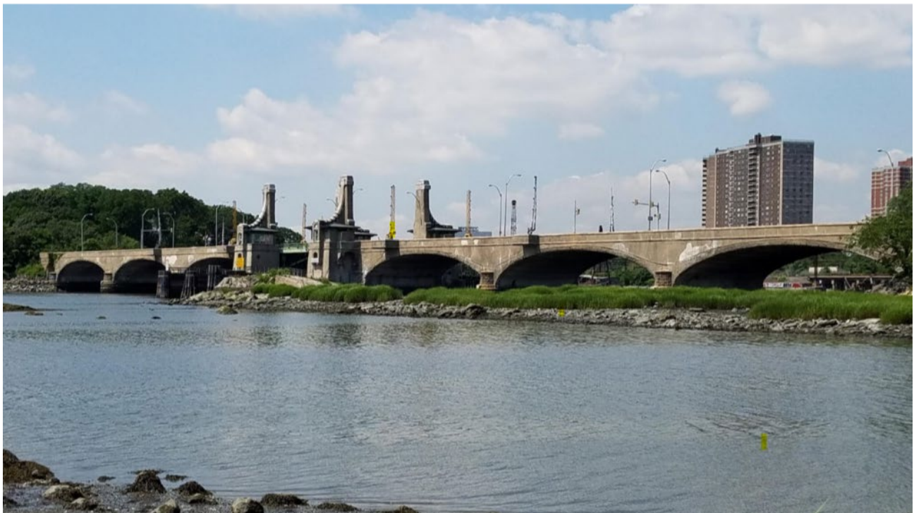
Figure 1. Shore Road Bridge (Source: NYCDOT)
