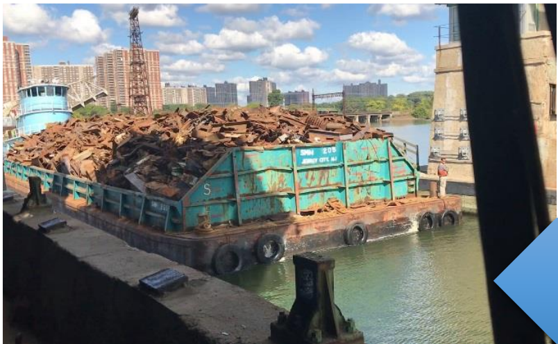
Barge In Narrow Bridge Channel
