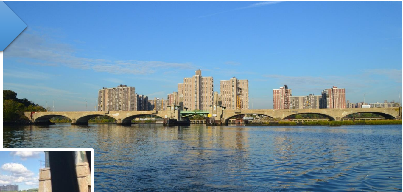
South Side of Bridge Looking North
