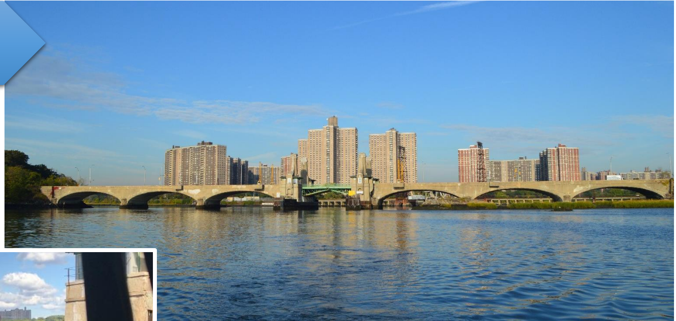
South Side of Bridge Looking North
